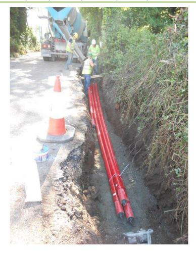
Plate 2-1: Cable Duct Laying in Trefoil Configuration
